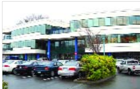
Dynamotive Energy Systems Corp. is headquartered in Vancouver, British Columbia, and has a plant in West Lorne, Ontario, and one under construction in Guelph, Ontario.
